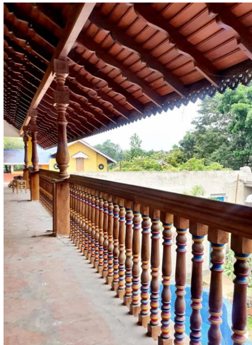
Upper-floor balcony and timber roof detailing
