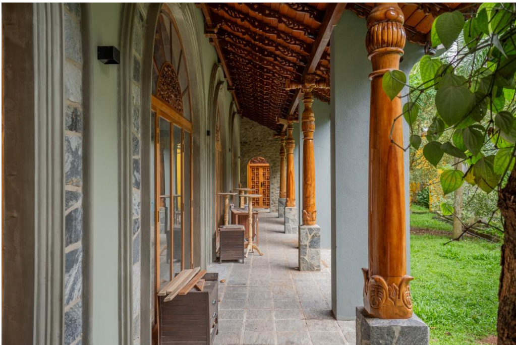
Timber columns and the ground-floor verandah
